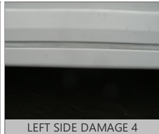
LEFT SIDE DAMAGE 4
